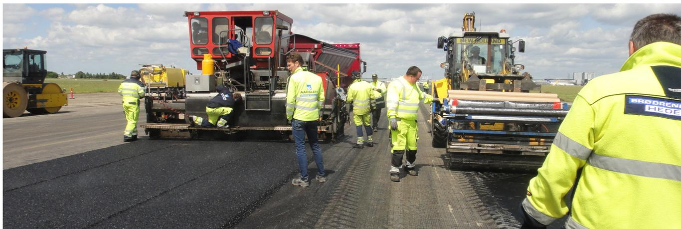
▲ Mechanical unrolling of S&P Carbophalt® G in one of the busiest areas of the airport and application of new asphalt pavement onto the S&P grid
